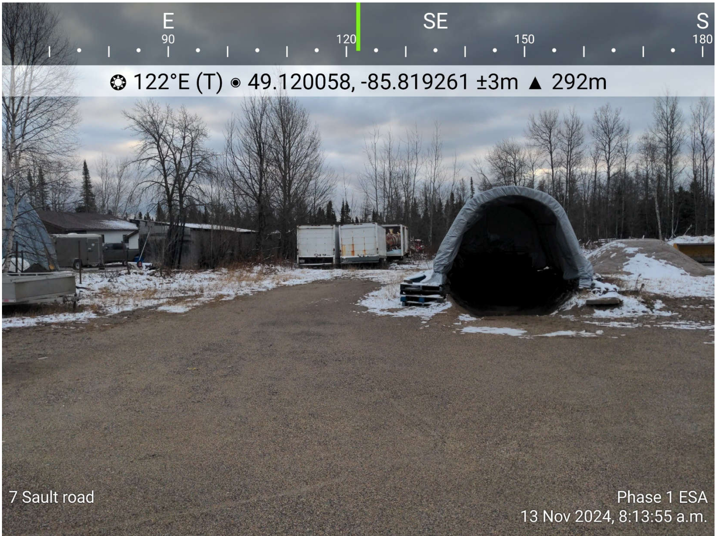
Photo 1: View facing southeast of the subject property.
