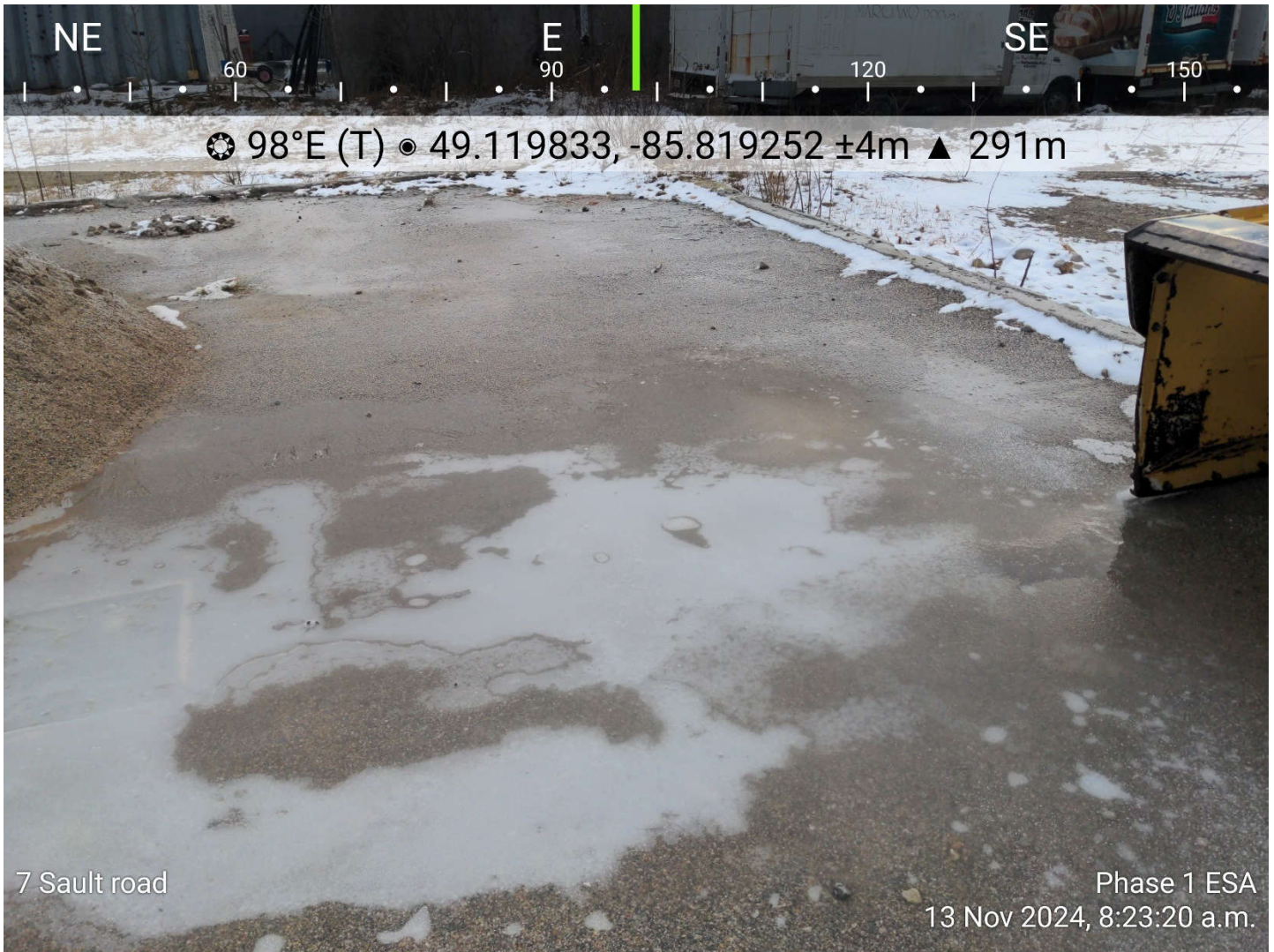
Photo 6: View facing east showing the concrete pad integrity.
